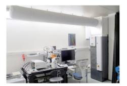
**Institute of Experimental Botany CAS**Laboratory of Confocal Microscopy – STULZ precision air-conditioning units, for optimal supply air distribution are used textile diffusors Clean room with close temperature control +/- 1 °C.
